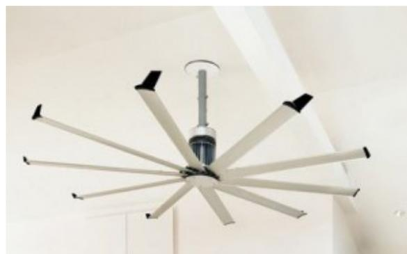
These winglets at the fan blade tips help to smoothen airflow around the fan blades which would lower drag and increase airflow. Also note the slanted fan blades (photo from [www.modenus.com](http://www.modenus.com)).
